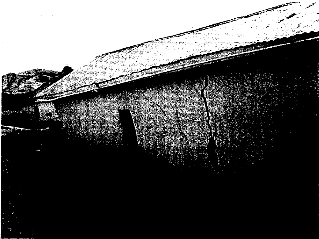
Storm damage has left building unstable.
